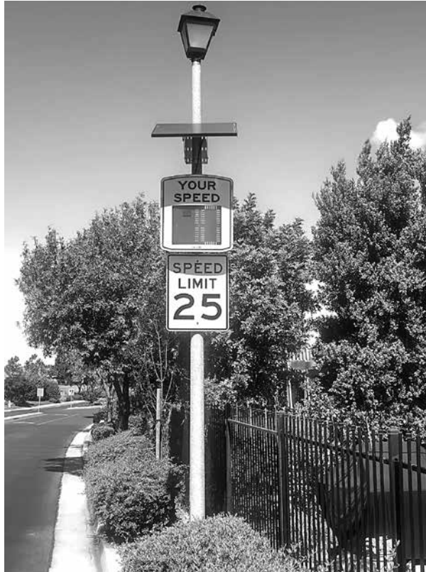
Speed monitor installed on Summerset Drive.
