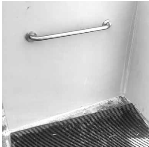
Recently installed grab bar at Delta Pool shower.
